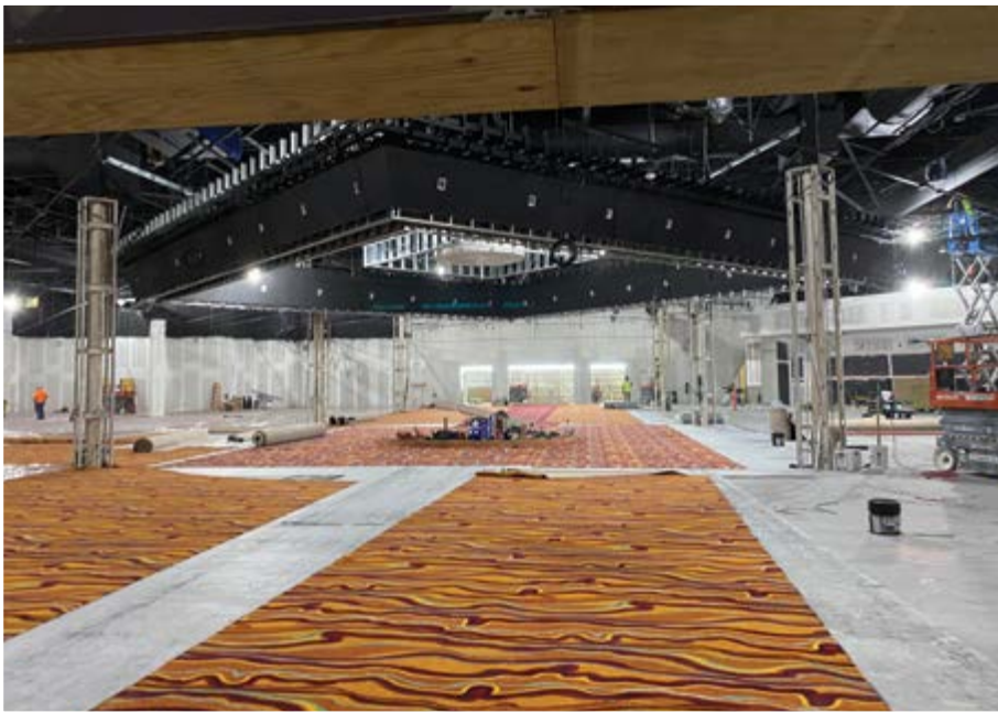
Construction continued on Parx Casino Shippensburg as the fiscal year concluded.
